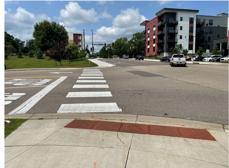
HyVee Entrance on 36 th Ave.
