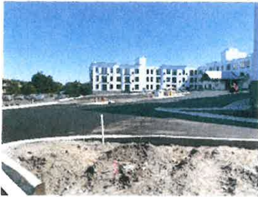
First lift of asphalt
