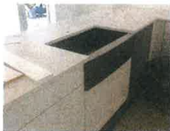
Unit kitchen sink
