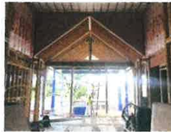
Main lobby framing and insulation
