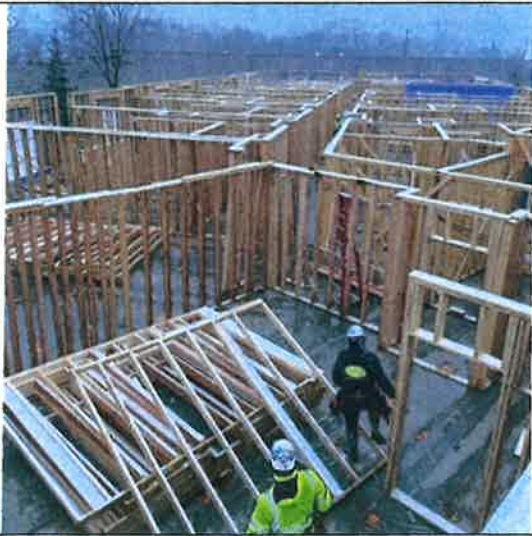
Zone 3 level 1 framing
