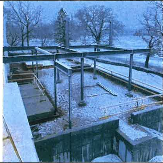
Zone 2 structural steel
