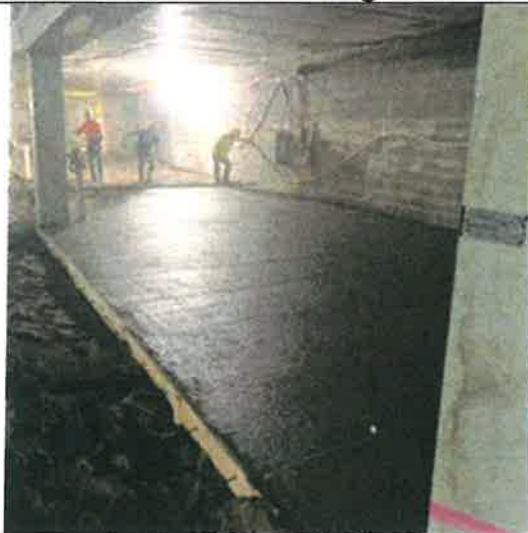
Garage slab on grade concrete
