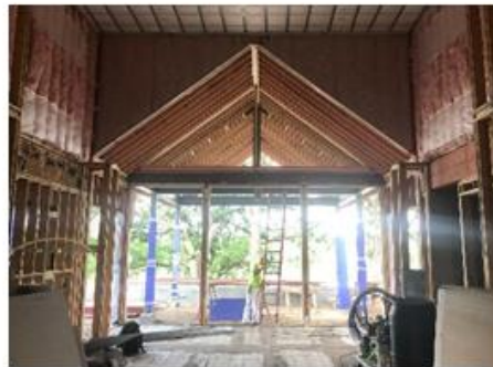
Main lobby framing and insulation
