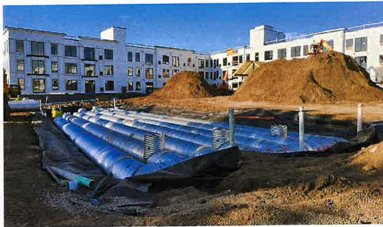
Underground infiltration system installation at The Reeve Lakeside Apartments on Lower Twin Lake - 6/8/2022
